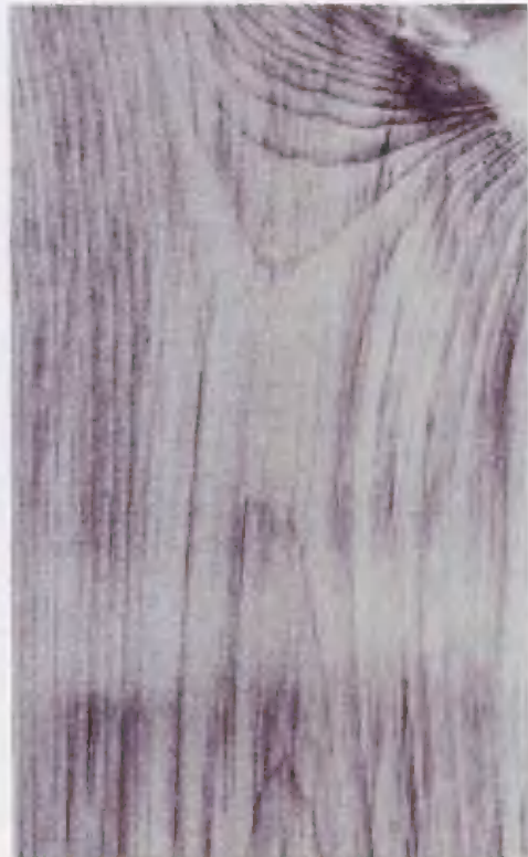
Brown stain: Brown color caused by a wood sugar/enzyme reaction to very high temperatures in kiln drying.
